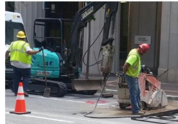
Worker using a walk-behind saw with an integrated water delivery system to cut asphalt roadway.
